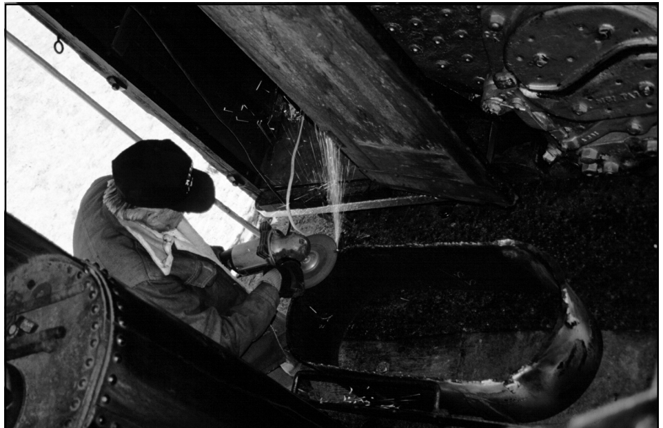
Ralph Vance grinding the tender water fill hatch.- Photo © Steve Mason
